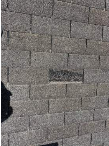
Roof, Missing or Broken Shingles
